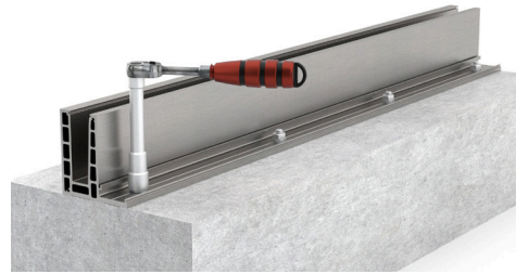
2. Place the profile and secure using a torque wrench set to 40 Nm.
