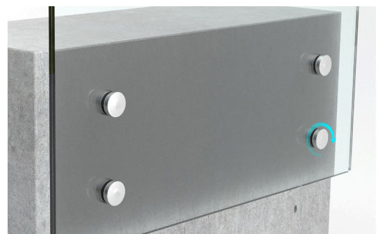
4. Once everything is in place screw on top part of the standoff. Finished look.
